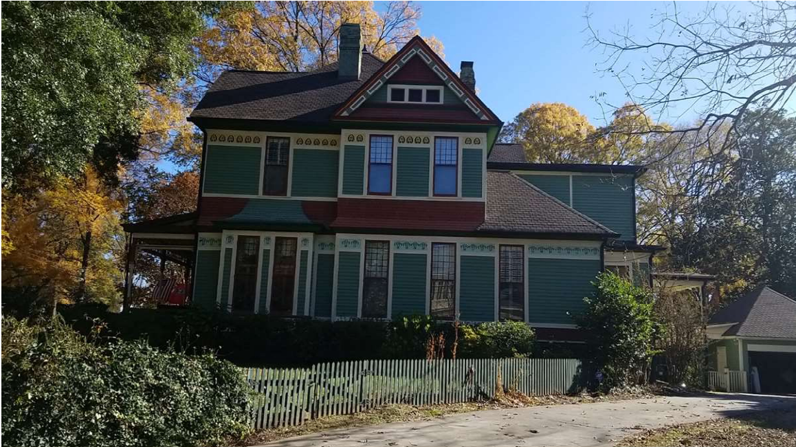
Existing House: View from Franklin
